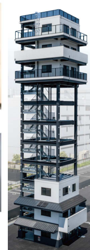
33m (11-story) Training tower
