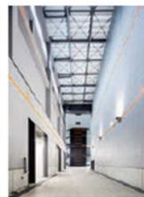
● Water Discharge Passage (55m)
