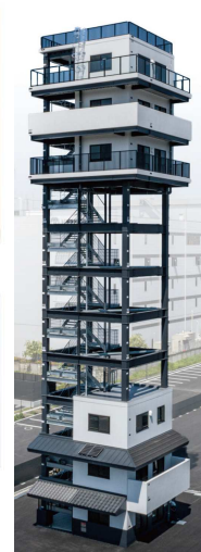
33m (11-story) Training tower
