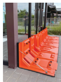
Quick flood barrier that can be easily installed to prevent flooding caused by torrential rain (Left: Side view, Right: Warehouse entrance)
