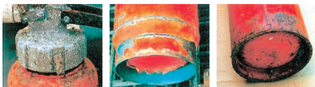
Badly corroded fire extinguishers
